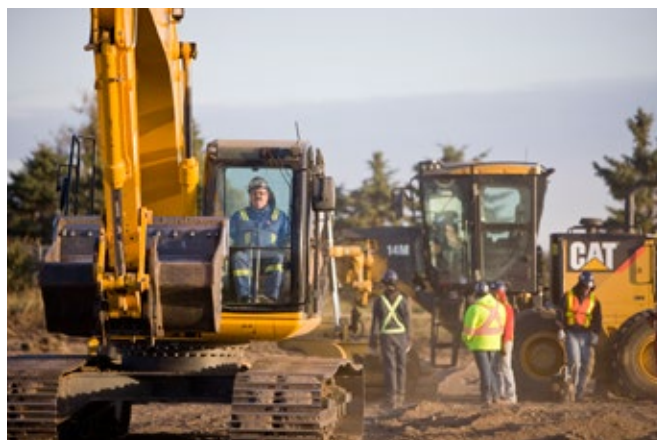
Heavy Equipment Operators in Action
